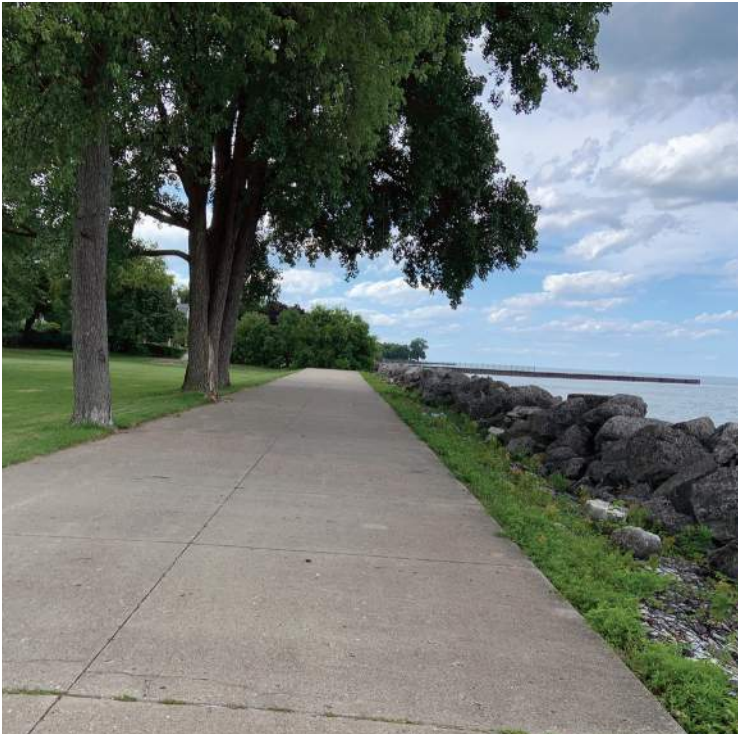
VIEW OF CONCRETE PROMENADE AND RUBBLEMOUND REVETMENT, LOOKING NORTH
