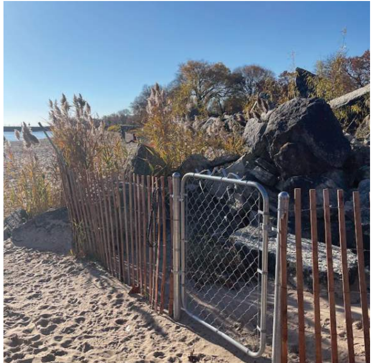
EXISTING LOWER GATE AT THE ENTRANCE TO DOG BEACH
